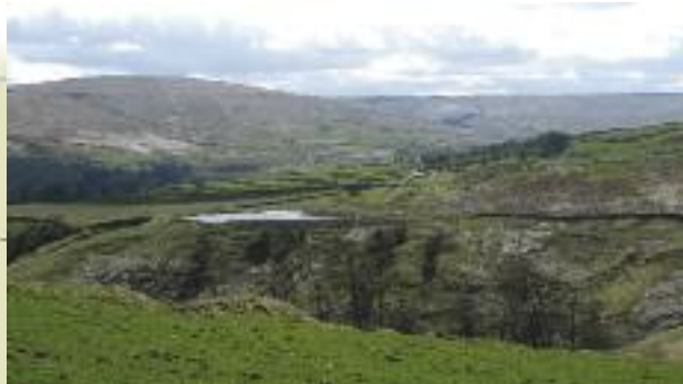
West Slitt dam and reservoir, with the line of the former railway crossing the slope
